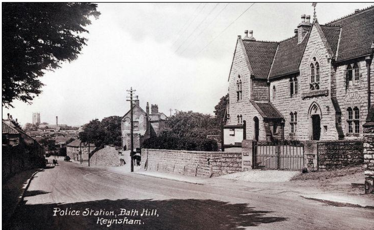
Fig. 2 Keynsham Police Station
