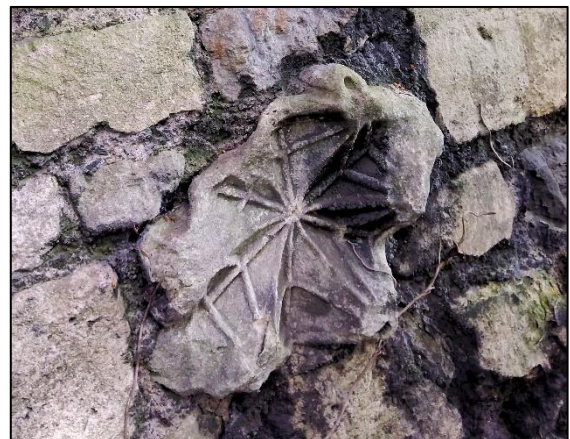
Fig. 9 Carving incorporated into the Park House arch by Mr Cox. Probably originally from the Bedford chantry chapel.
