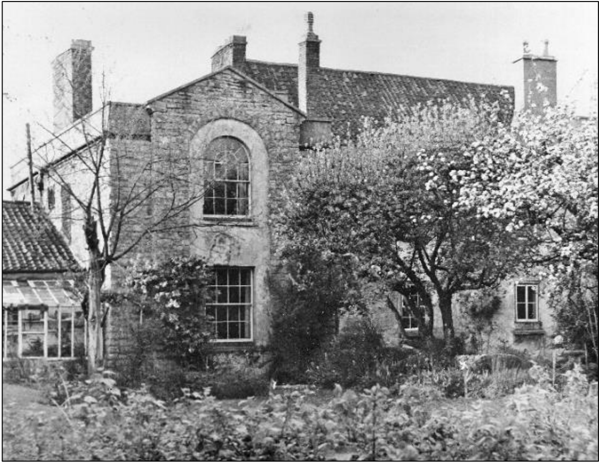
Fig. 5 Rear view of Flanders House.
