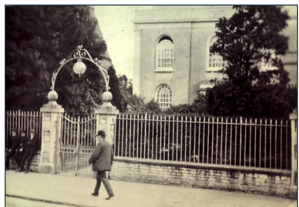
Fig. 2 Front of Keynsham Baptist Church before the railings were removed.
